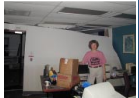
Deborah Halsted Surveys Damage in the NN/LM SCR Offices
