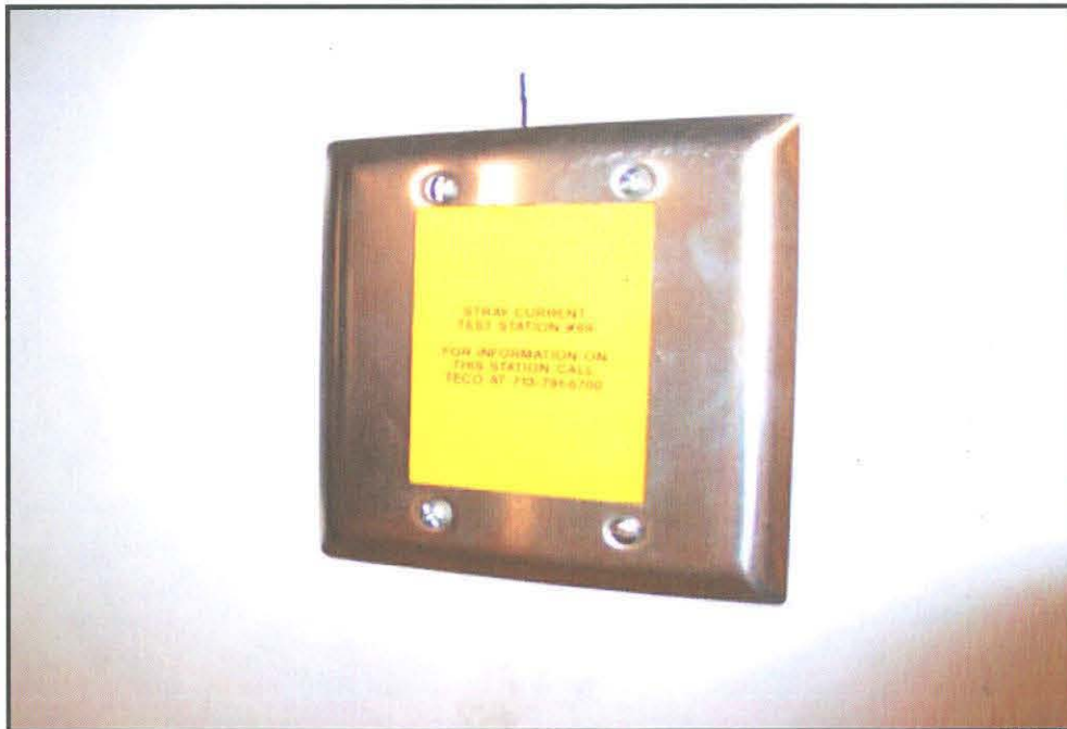
b) TECO-Installed Wall Plate Over Test Connection
